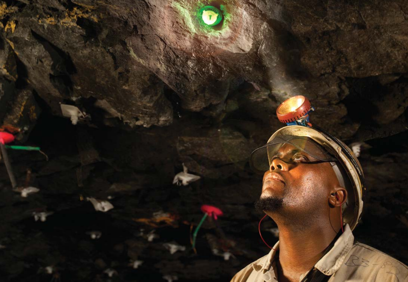
Sydney Mabale observes a fall-of-ground light installed to monitor ground movement
