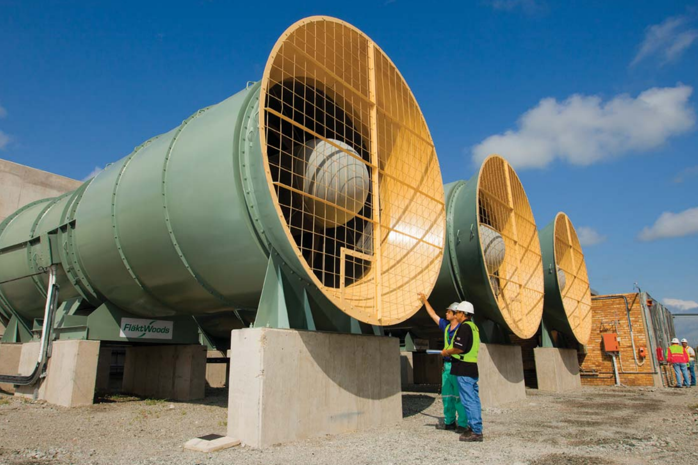
Willie Pienaar and Pierre Hattingh discuss commissioning of the new refrigeration plant at Khuseleka Mine
